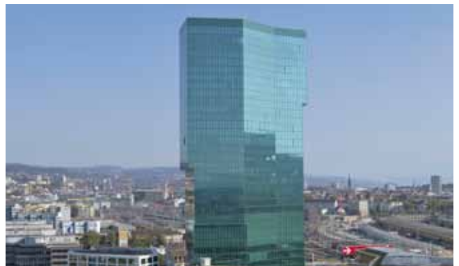
Prime Tower, Zürich
